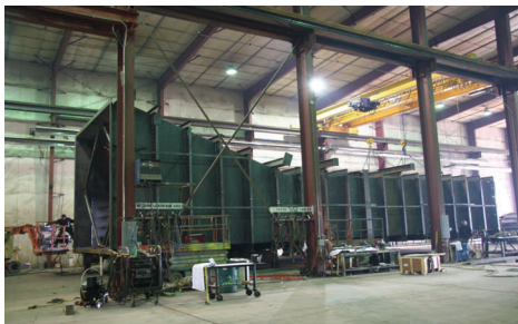
To the Left is the Ductwork Project Bill Hartig is working on.
