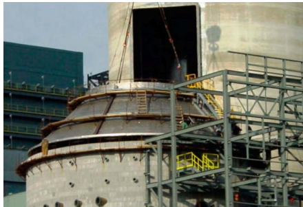
Absorber hood and tower system
